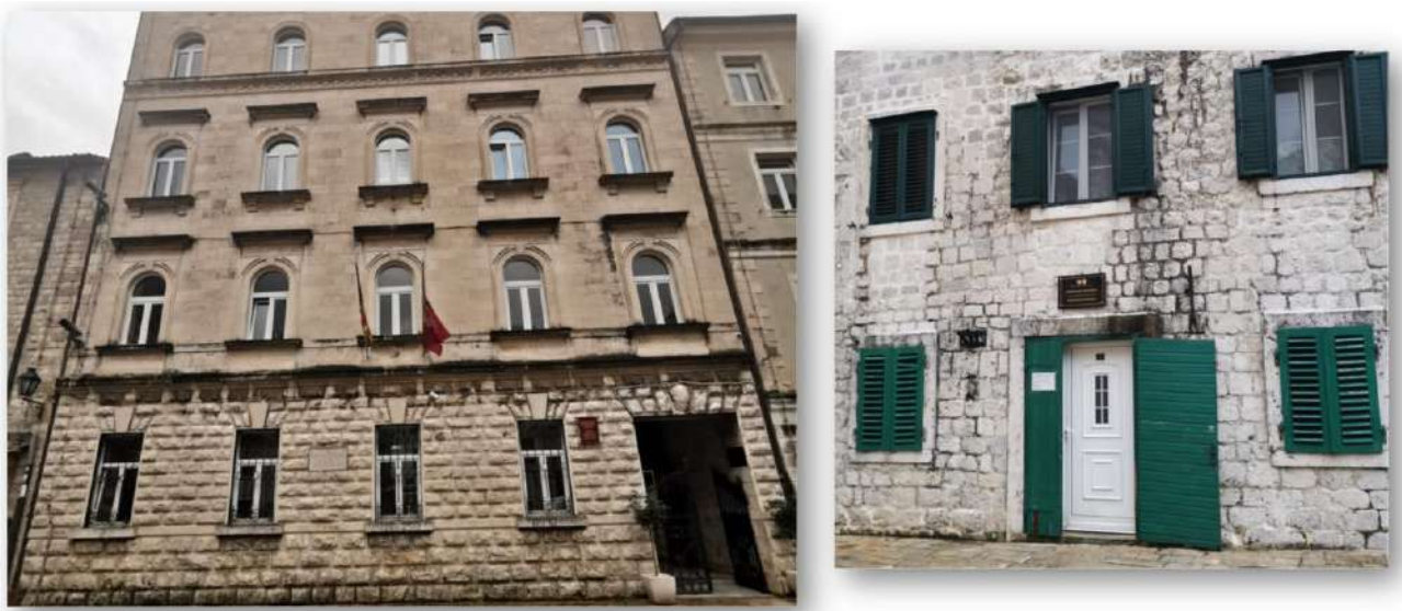
Figure 43 : An example of possible improper building facelifts in Kotor Old City
