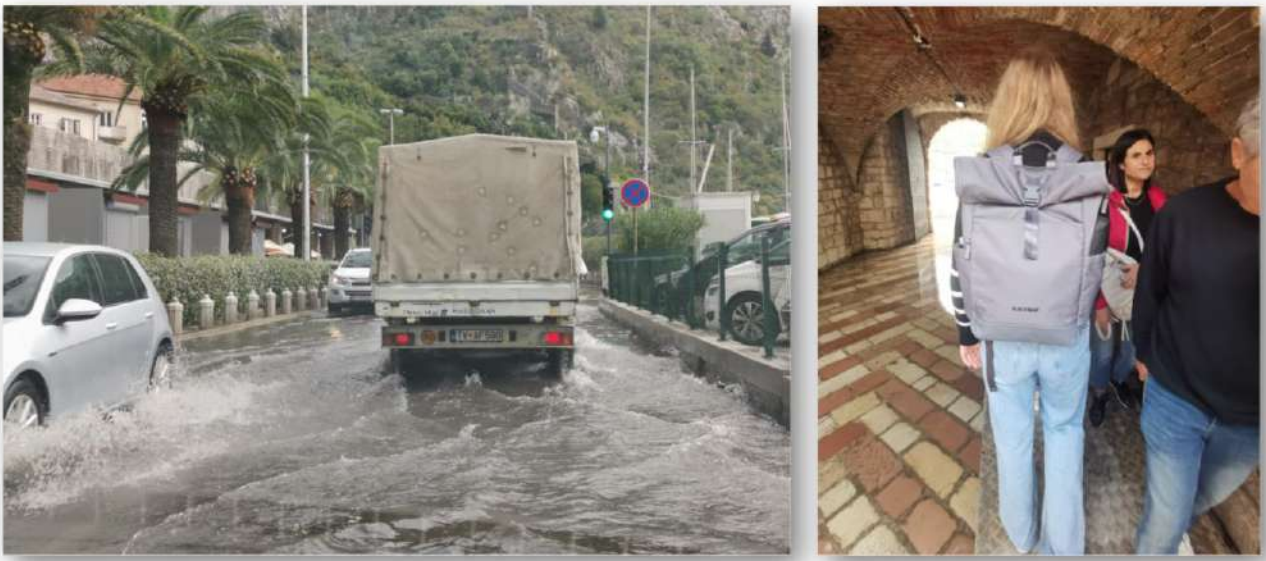
Figure 50 : An often example of sewage management issues in the old city gates
