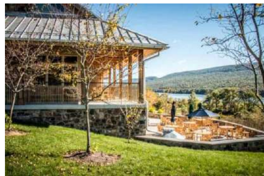
The Nature Inn at Bald Eagle State Park incorporates Design Guide principles of green technology and local artisan products into its building design. [Photo courtesy of PA Wilds Center for Entrepreneurship Inc.]
