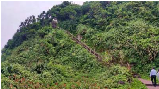
Rebuilt stairways can handle increased foot traffic to the peak. Photo Credit: Roi Ariel
